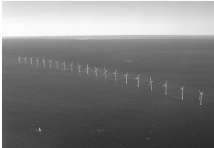
20 turbines, rated at 2 MW each, in Denmark's Middelgrunden Offshore Wind Farm. Photo © BONUS Energy A/S.
